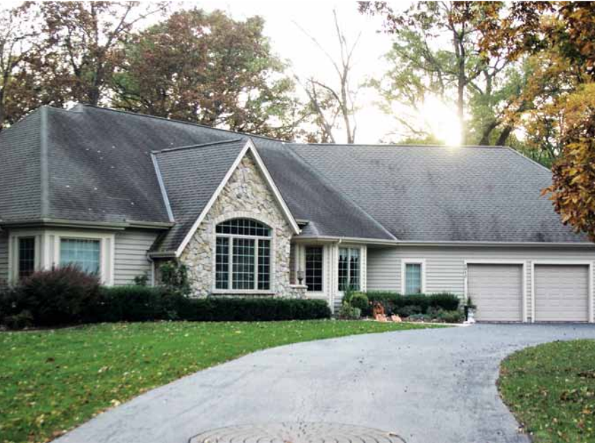
Stains are visible across the rooftop.
