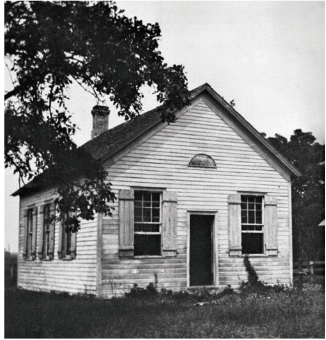
The Porter Schoolhouse in the 1890s. It was a balloon frame one-room school, on Porter, now Buckley Road. ( Tales of Old Barrington )
