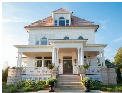
Above: The Julia and John Robertson home as it appeared in 1904. Below: The Robertson Home was placed on the National Register of Historic Places and preserved as Barrington's White House.
